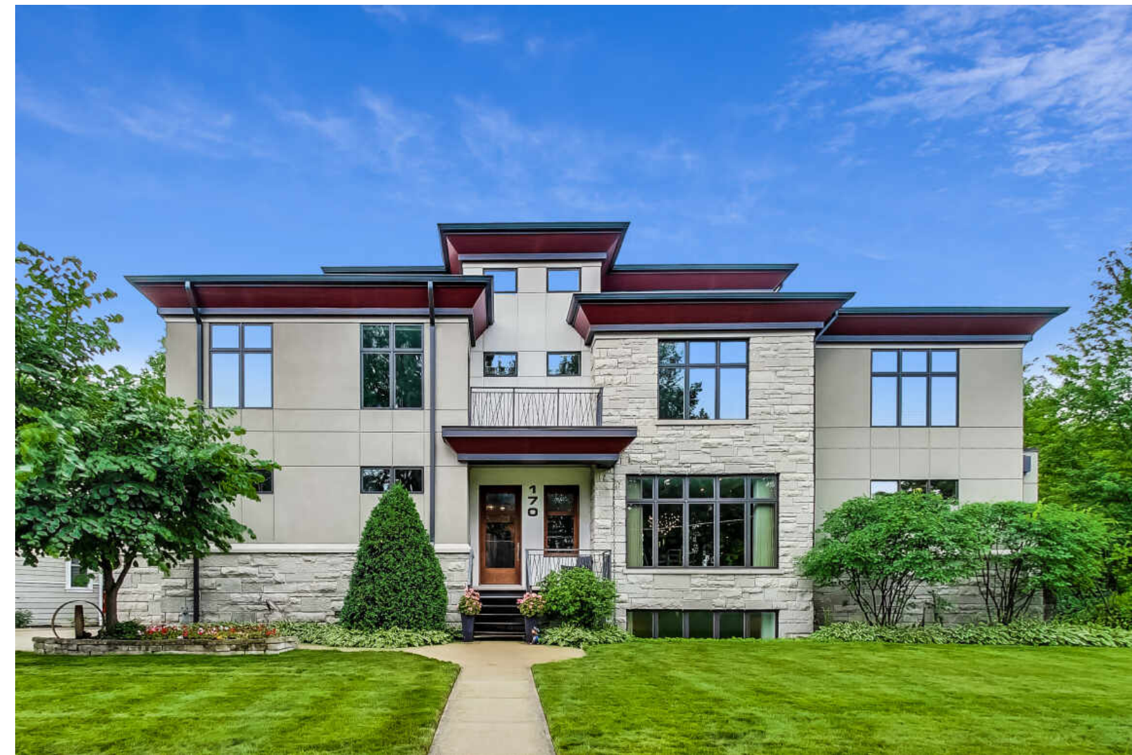
170 E SOUTH STREET • ELMHURST
