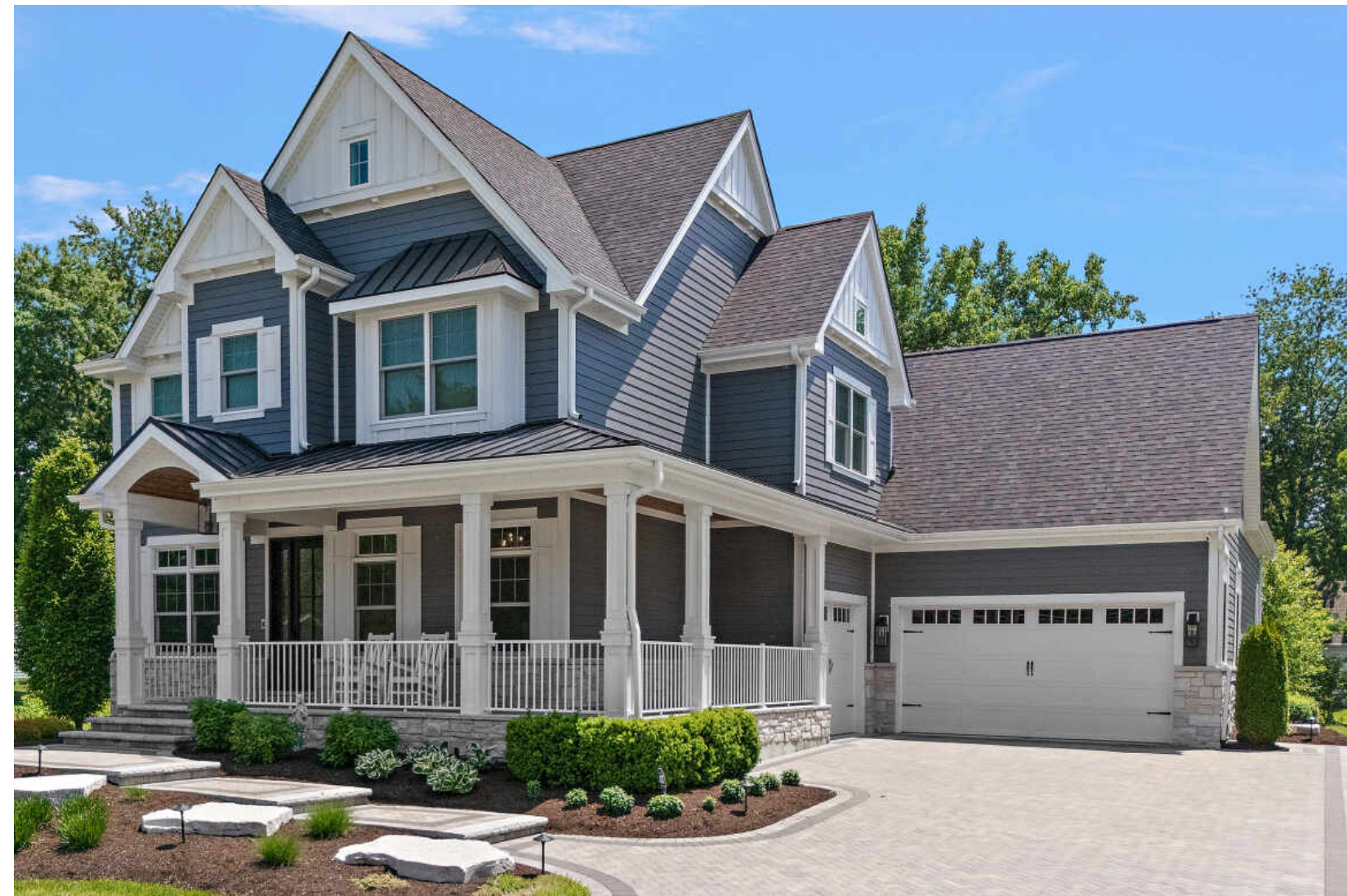
306 NEBRASKA STREET FRANKFORT
